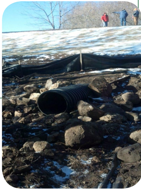
Above: A pipe coming out of the berm controls the rate at which runoff discharges to the gully below.
