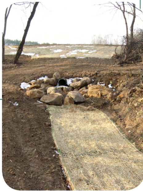
Above: An outlet structure and erosion control materials prevent runoff from causing further erosion.
