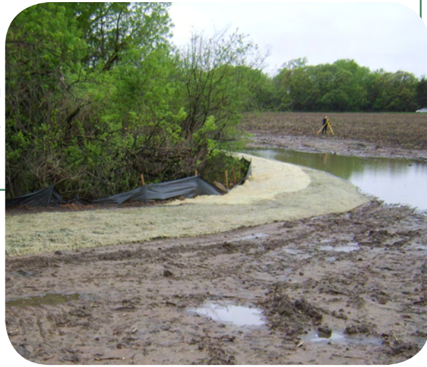
Above: Runoff water from rain and melting snow pond behind the berm instead of flowing straight into a gully in the woods.
