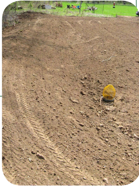
Above: The newly constructed berm and rate control structure before seeding.
