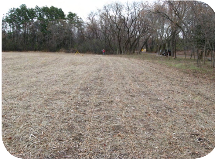
Above: Surveying the field before building the sediment basin.
